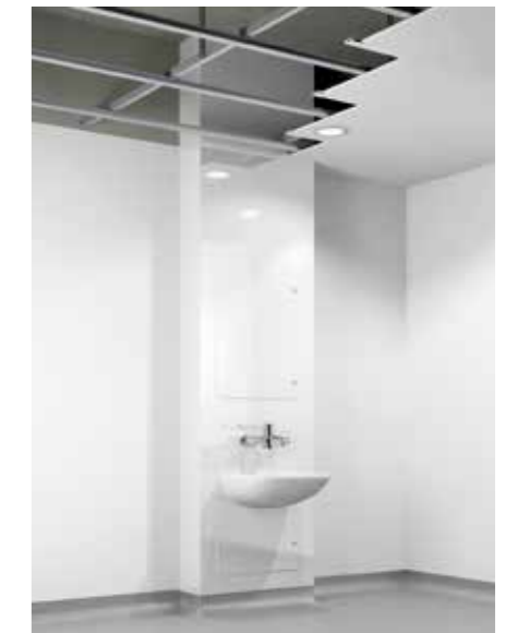
Through suspended ceiling
