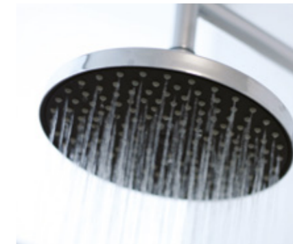
Showers and washrooms
